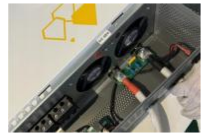
Inverter positive and negative pole installation completed status
